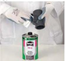
It is advisable to use an applicator/brush of dimension not less than half the diameter of the pipe. The solvent cement must be applied along the entire length of the joining surface of both the pipe and the fitting:
